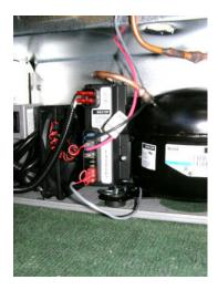
Photo shows unit wired for low speed. Thermostat is on C-red, P-red, T-black
