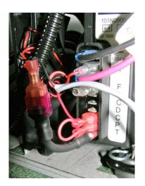
Photo shows unit wired with speed resistor in series with thermostat wire and reconnected to T
