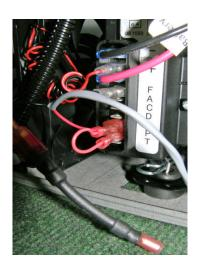
Photo shows unit resistor on black thermostat wire and ready to be put back on the T spade on the bottom of the module. This is a medium speed resistor shown in black shrink wrap. Red shrink is a high speed resistor.
