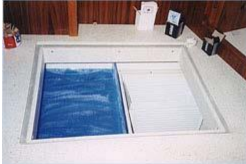
Shows Nova Kool RT6 mounted near the top of the freezer section.
